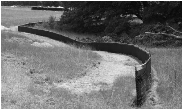
Pictured above is an example of silt fence installation used to prevent sediment and debris from flowing off a construction site into streams and waterways during storms.
